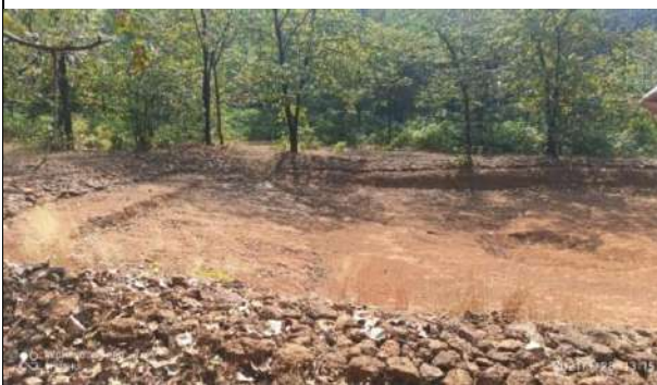
Dry stone pitching for Cumari water pond
